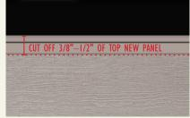
Push the new panel of siding up and under the good siding piece above it and then push and/or bump the new panel down until it locks down on the good siding panel below it.
