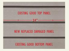
6 To secure the upper good panel and the new replacement panel install 1-3/4" stainless still ring shank trim nails and pound in with a small hammer being careful to leave the back head of the trim nails 1/16" from tight. This allows for outward heat expansion of the two panels.
